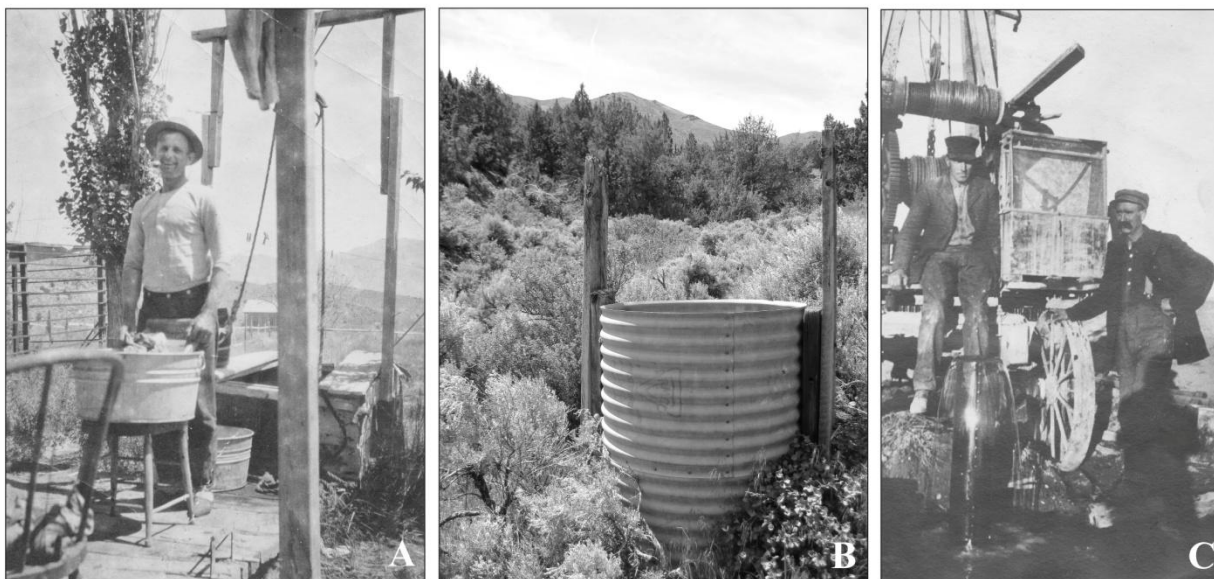
Figure 4-7. Water wells in Kennedy. (A) Bill Zuick doing his laundry in front of a rope-and-bucket well. Zuick lived in the Benton house (1-6, Fig. 4-2B); a deep hole at this general location was the well hole. Taken in the late 1910s or early 1920s. (B) Culvert pipe in gravels next to Kennedy Creek near the Crown Point (Sunnyside) mine (Fig. 4-4). The vertical wooden boards held a cross bar from which a bucket was suspended, similar to (A). The well provided abundant fresh, cold water in 1976. (C) Charley Kennedy (right) and an unidentified man using a wagon-mounted Keystone water drilling machine in Kennedy. Probably taken in the mid 1910s. Abundant water was flowing out of the drill pipe in the left foreground. Sources: (A), (C): the Stanley McCoy collection; (B) photograph by the author.
