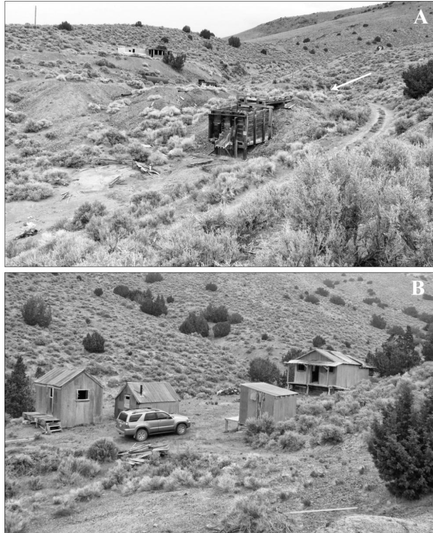
Figure 7-7. Henrietta mine area today. (A) Photograph of the lower tunnel area of the Henrietta mine area, showing the ore bin, mine tailings, and buildings at the mouth of the lower tunnel (Fig. 7-2). The white arrow points to the tunnel portal; ore-cart rails extend to the top of the ore bin. The small light-colored area to the lower left of the ore bin may have been the site of the later mill. The building in the upper left is a mobile home of younger vintage. (B) Buildings constructed for mine workers in the late 1920s. The left and right buildings have small cooking areas; the middle building behind the truck was for sleeping; and the front building was a shed. Taken by the author in May 2013.
