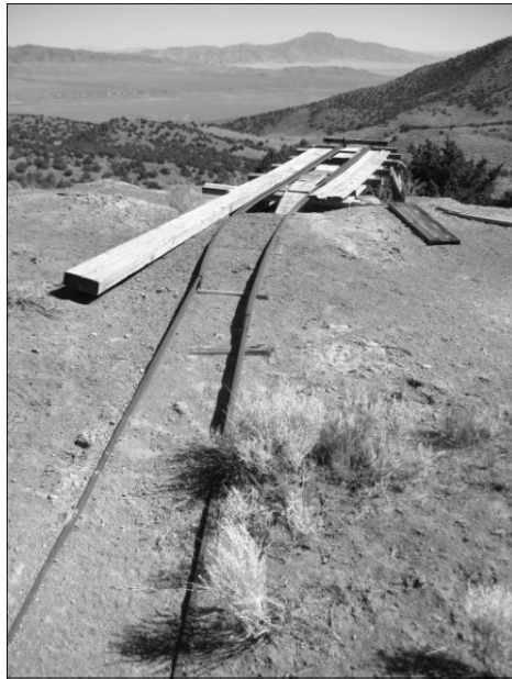
Figure 3-11. Ore-cart rails leading from the mine to the loading platform in the background, Black Hawk (Cricket) mine. These features likely date back to the 1930s, during Clark Ringling's ownership of the mine. Photograph taken in 2010.
